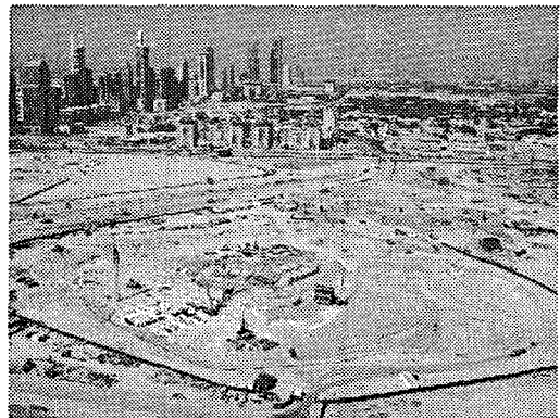
Figure 10: Burj Dubai Site as of March 2005
