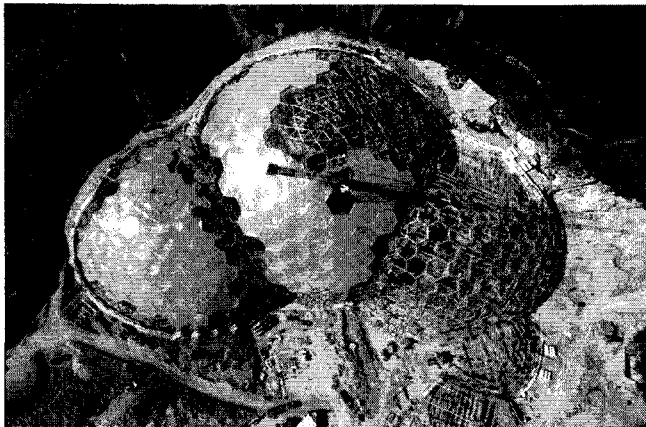
Fig. 17 Erection of the HTBiomes
