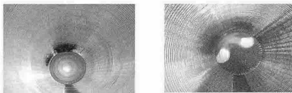
(c) Before removing scale of the outlet
