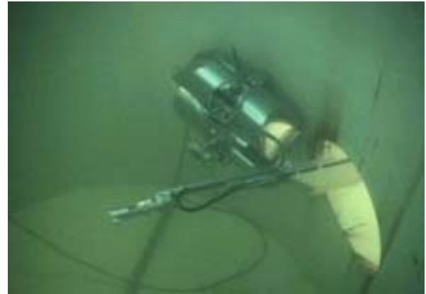
Fig. 8 Inspection of nozzle welds
