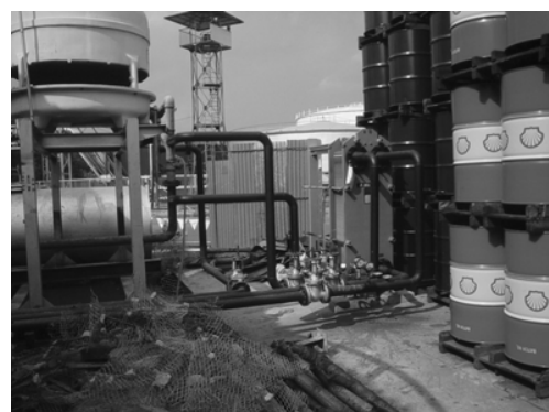
(c) After plate heat exchanger installation Fig. 5 Cooling system improving.
