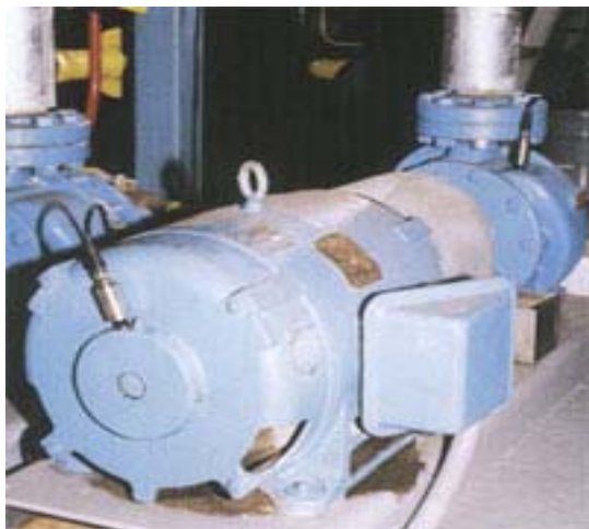
Fig.2 ultrasonic signal measuring method in site
