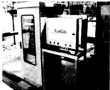
Figure 5. DAS & Oil monitoring system in Yeosu T. P.
