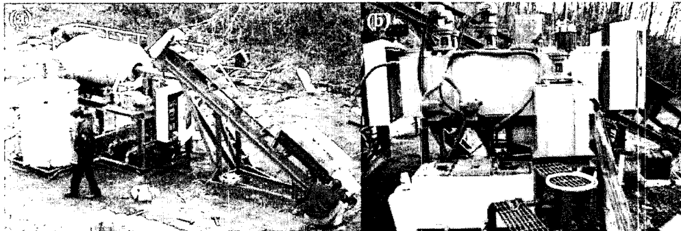
(a) soil washing system
