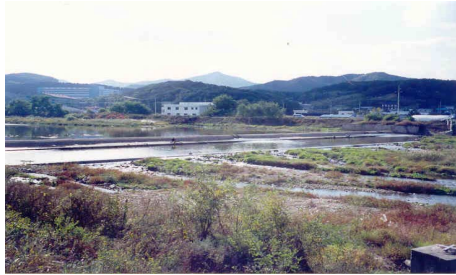
Fig. 1 Before removing a low dam
