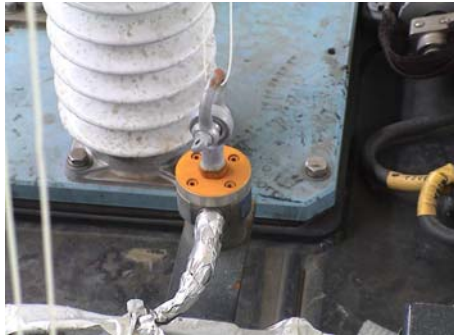
Fig. 6 Lift load cell on the roof
