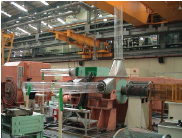
Photo. 1 Generator fan & experimental device
