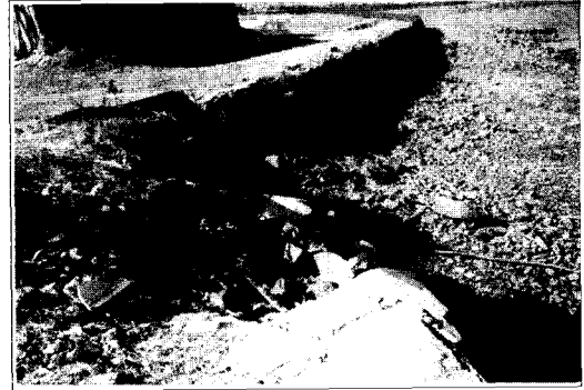
Fig. 5. Example of seawall collapse.
