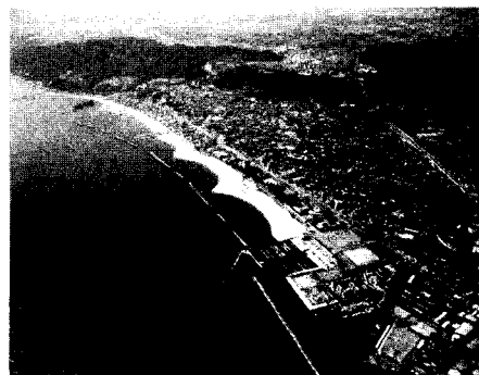
Fig. 2. Suma artificial beach applied environmental windows (Kobe City, 1990).
