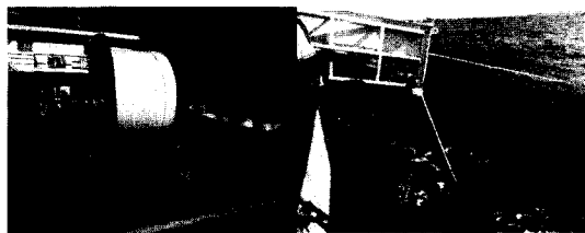
(3) Cable Dram (4) Edge of the Barge
