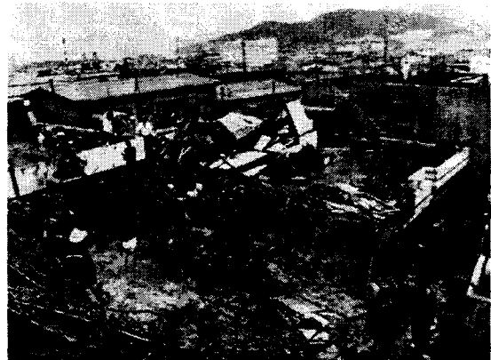
Figure 6. Landslide damage to private houses due to the heavy rain.
