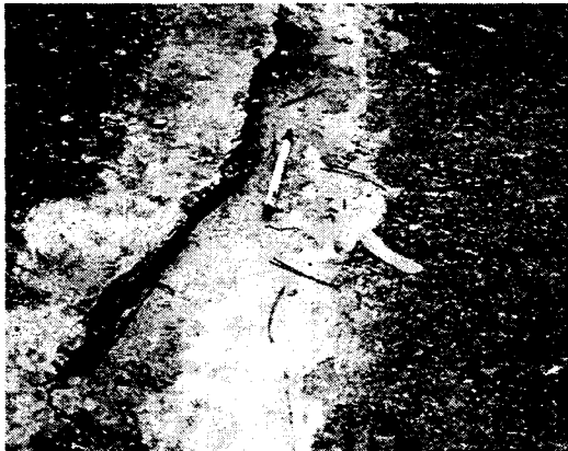
Figure 5. Curved tension crack in the foreground.
