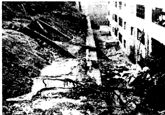
Figure 4. Landslide damage to the Sangah apartment.
