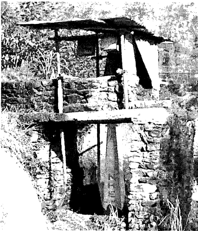
Fig. 2. 200W hydro power used for village electrification.
