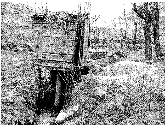
Fig. 1. 200W picohydro generator used for village lighting with white LEDs.
