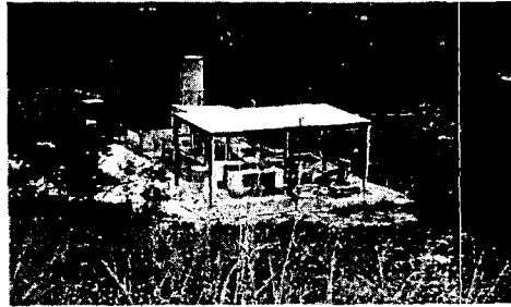
Fig. 2. Overview of Landfill Gas to Electricity Facility at the Jordan Valley Landfill
