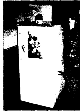
Fig. 2 Gas Vent Box
