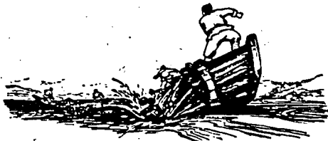
Fig.45 Dumping of rubbles from boats
