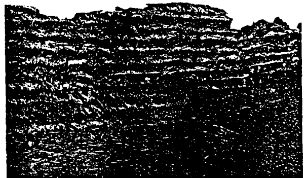
Fig.27 Loess wall reinforced with twigs and reeds
