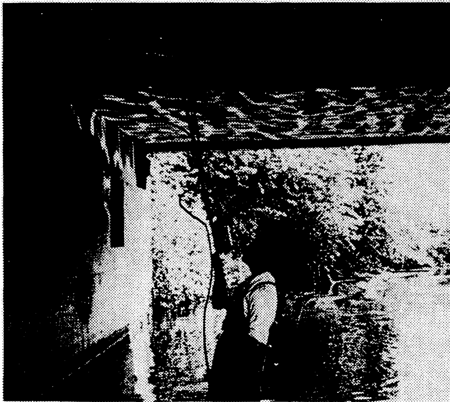
Fig 11.- Portable, hand held, Ground Penetration Radar ( GPR ) for structural survey under a reinforced concrete bridge.
